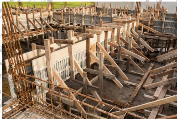
Gambar 2. 1 Bekisting konvensional
