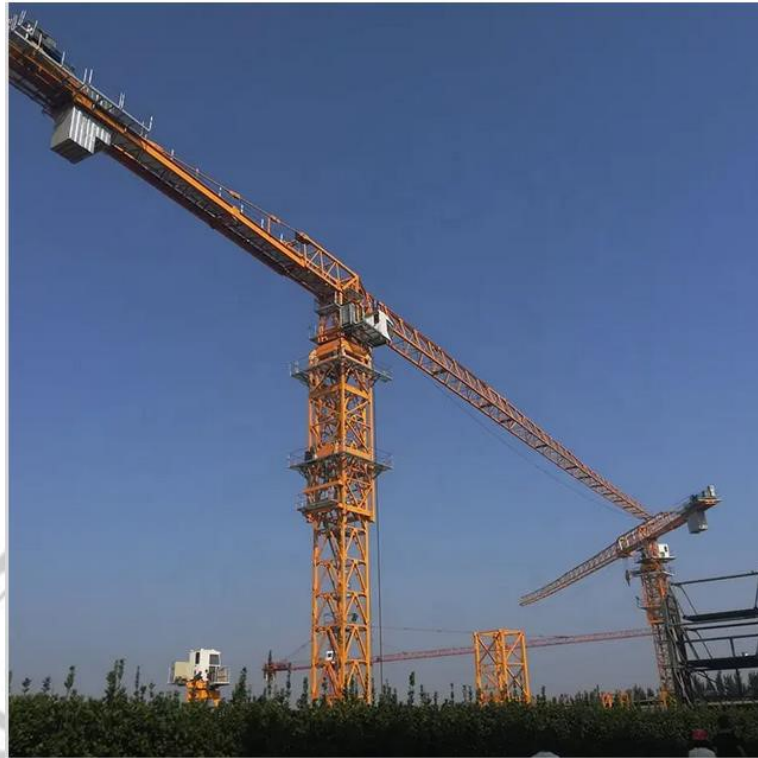
Gambar 2. 3 Tower Crane ZOOMLION TC 6520-10E
