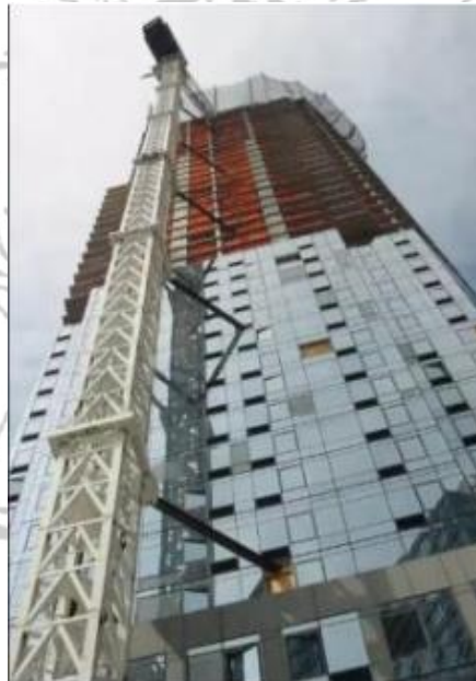
Gambar 2.5 Tied in Crane
