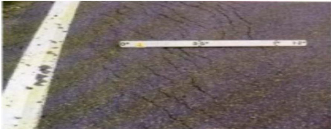
Gambar 2.18 Patah Slip
