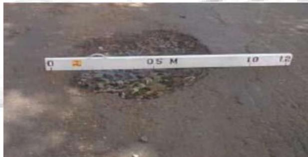
Gambar 2. 22 Lubang (*Potholes*)
