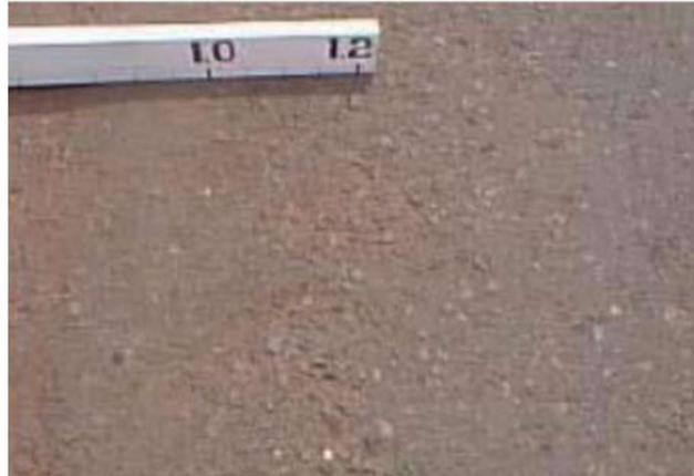
*Gambar 2. 24 Pengausan (Polished Agregate)*
