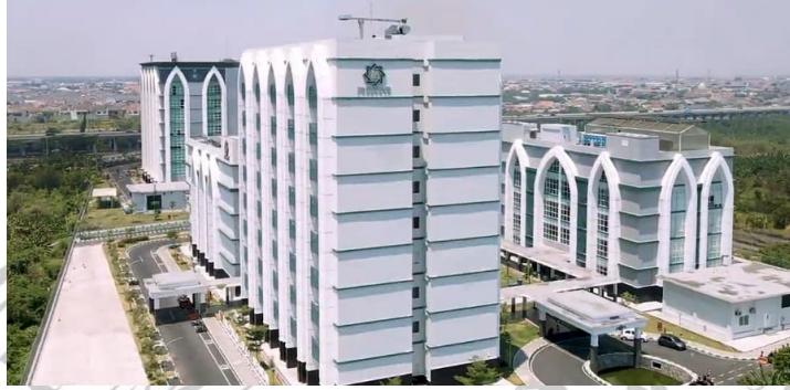
Gambar 3.1 Footage Gedung FPK UINSA
